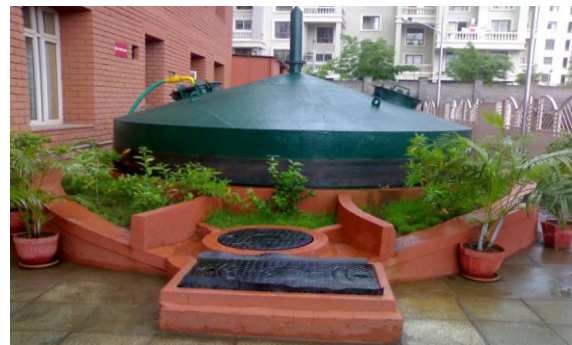
Bio digester of cow dung to produce bio gas as fuel
